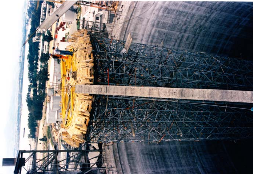
PPRESTRESSED CLINKER SILO (Ø40m) CONICAL ROOF PRECAST BEAMS, PRECAST SLAB ELEMENTS PILES FOUNDATION CONSTRUCTION 1996 HALYPS CEMENT S.A. ASPROPYRGOS - ATTICA
