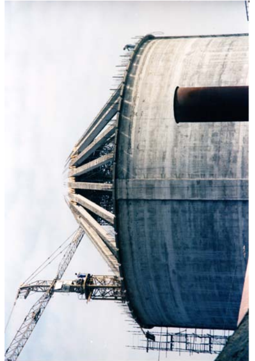
PPRESTRESSED CLINKER SILO (Ø40m) CONICAL ROOF PRECAST BEAMS, PRECAST SLAB ELEMENTS PILES FOUNDATION CONSTRUCTION 1996 HALYPS CEMENT S.A. ASPROPYRGOS - ATTICA
