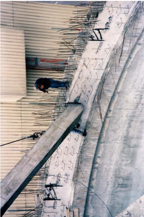
PPRESTRESSED CLINKER SILO (Ø40m) CONICAL ROOF PRECAST BEAMS, PRECAST SLAB ELEMENTS PILES FOUNDATION CONSTRUCTION 1996 HALYPS CEMENT S.A. ASPROPYRGOS - ATTICA
